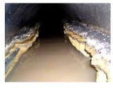
The city is having problems with grease building up and blocking pipes and the wet well. When this happens we are forced to hire a pump truck to come and
